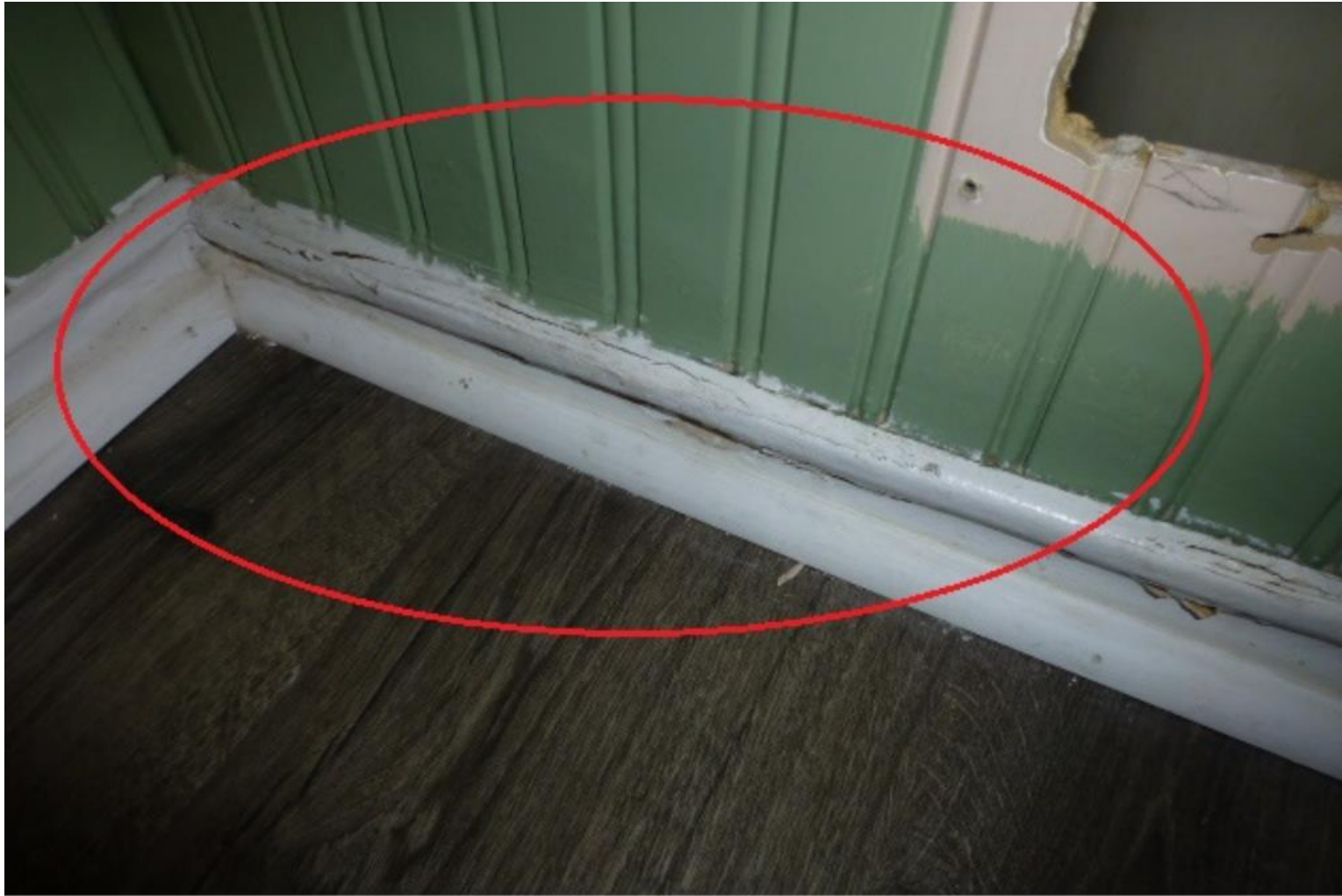
Moisture damage trim and wall in hall area
