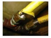
Trimming the protective outer jacket back too far exposed tubing should not be visible
