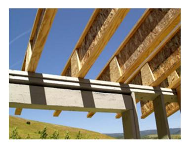
Web Stiffeners Generally Increase the Reaction Capacity of I-Joists.
