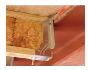
Flush bearing plate required. Maximum ¼" overhang permitted at beam.
